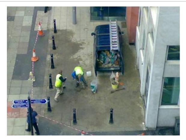
These contractors are installing steel pillars in concrete to stop vehicles from parking on the pavement outside a Sports Bar downtown. They are now in the process of cleaning up at the end
